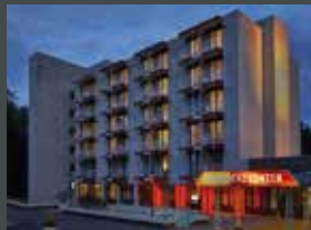
→ Hotel+ Hotel, Bad Soden/Frankfurt
